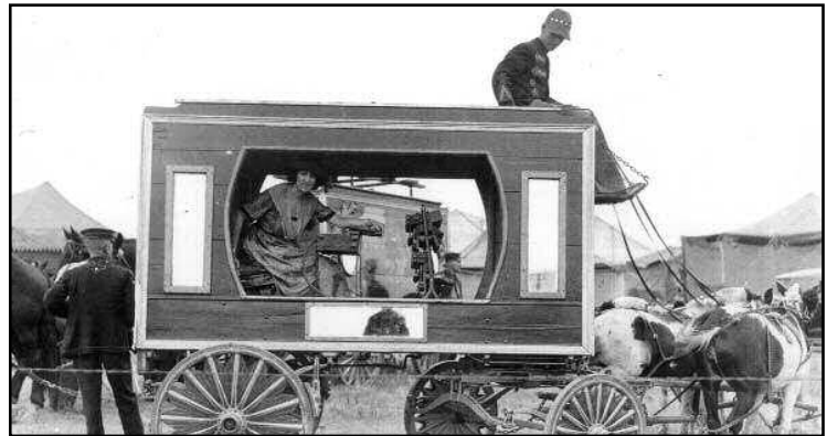
Figure 60. This view of the 1922 Gentry Bros. Unafon Wagon clearly shows how three levels of units could be made more compact by placing two at the same level, on either side of the rack. One hopes that the player wore ear plugs to preserve her hearing. Author’s collection.
